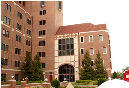
College of Social Work University Center, Building C
