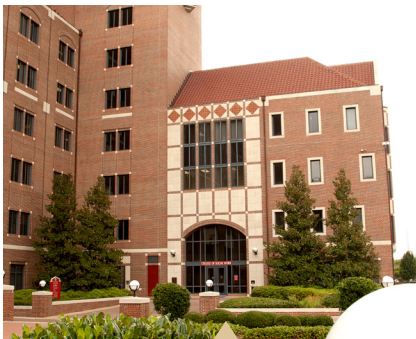
College of Social Work University Center, Building C
