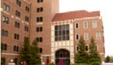
College of Social Work University Center, Building C
