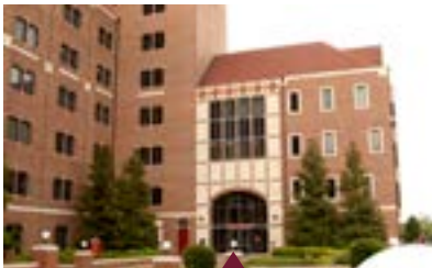
College of Social Work University Center, Building C
